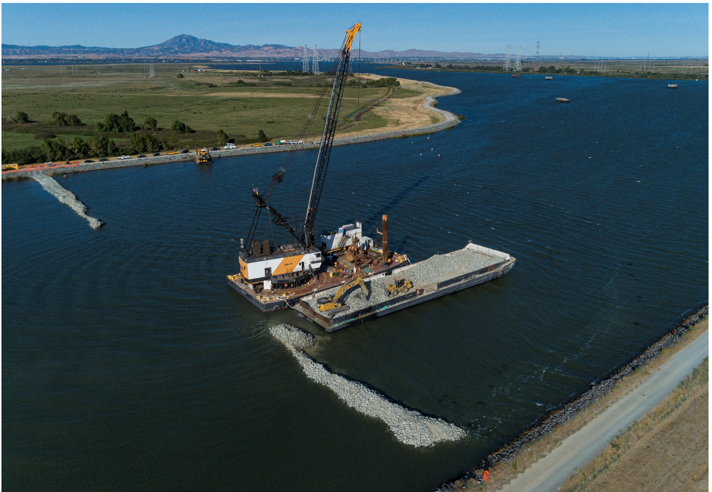
Installation of the emergency salinity drought barrier in the West False River (Photo: California Department of Water Resources)
